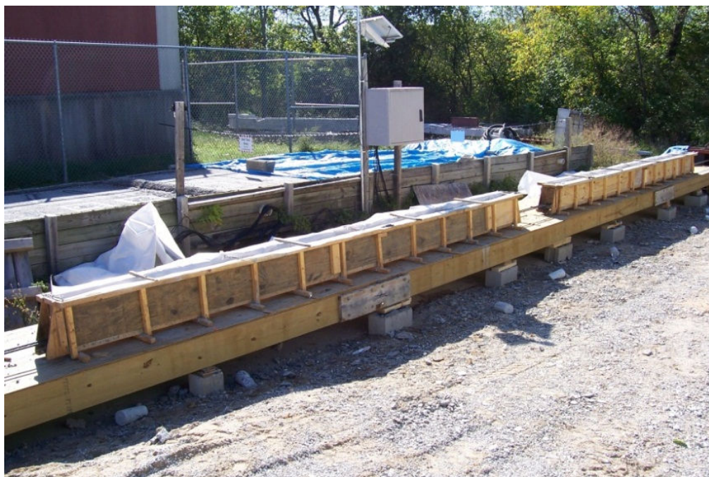
Figure 3.6 Beam Formwork
