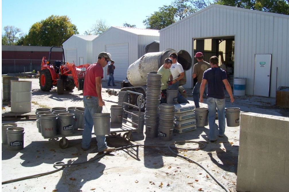
Figure 3.3 Loading the Mixer
